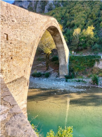
the bridge of Konitsa
